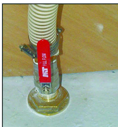
Thru-hull fitting open
